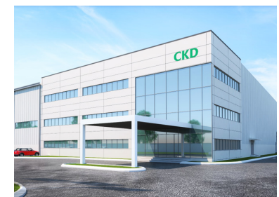
Indian plant (operational in 2023)
