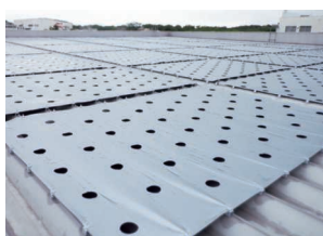
Installation of heat-shielding sheets (CKD NIKKI DENSO)
